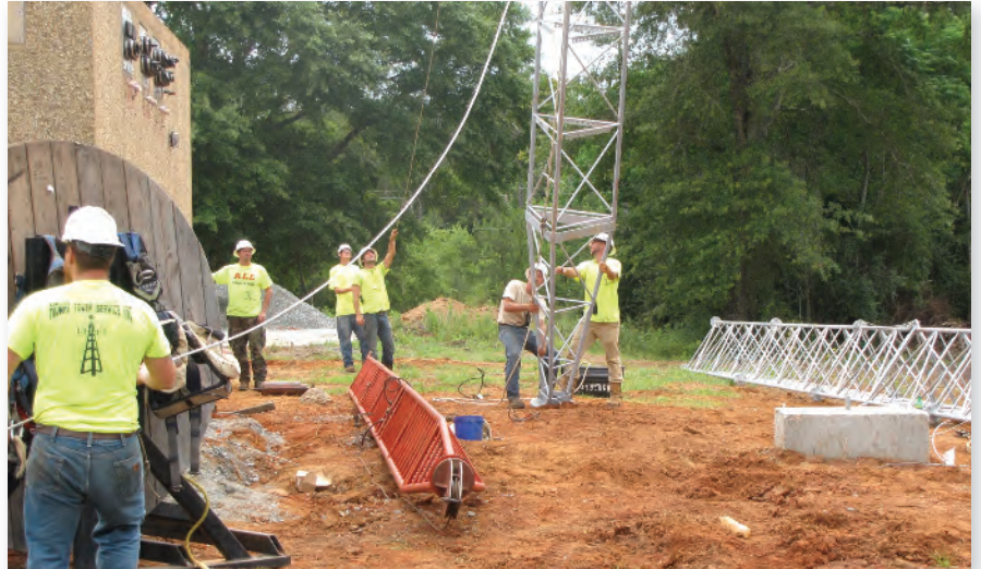
Tower construction crew contractors set the first section into place at this Cuthbert site.
