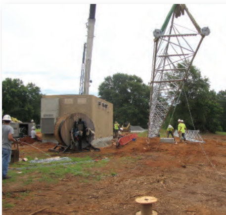
Using a crane, the tower construction crew hoists the first section of tower into place. Sections are added, one by one, until the tower is complete.
