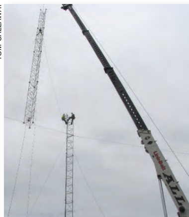
Using a crane, the tower construction crew hoists the first section of tower into place. Sections are added, one by one, until the tower is complete.
